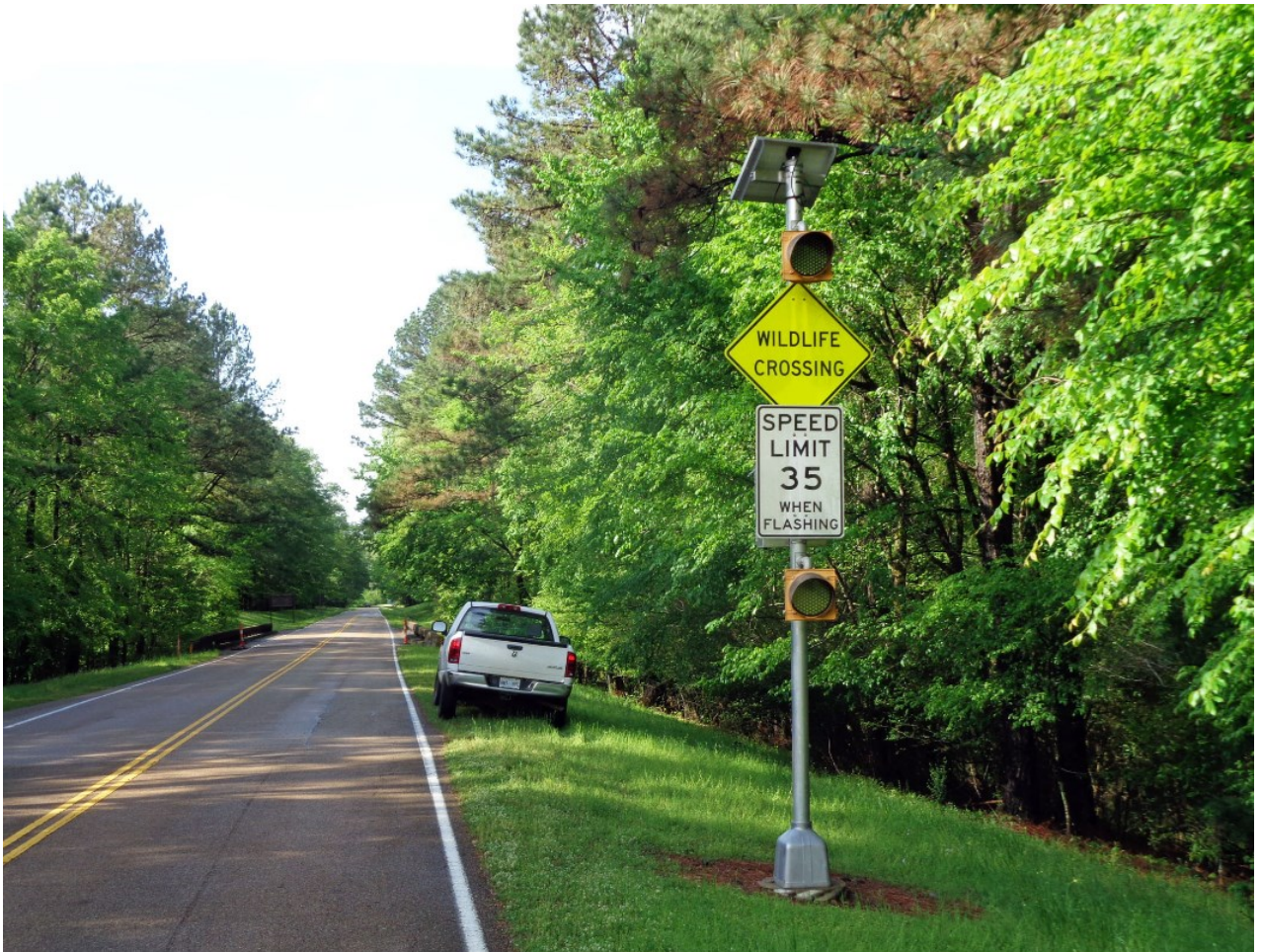
Figure 1. Solar/battery powered warning lights at wildlife crossing on the shoulder of the south-bound lane of the Natchez Trace Parkway just south of Interstate 20 in Clinton, Mississippi. Picture taken on April 3, 2017.
